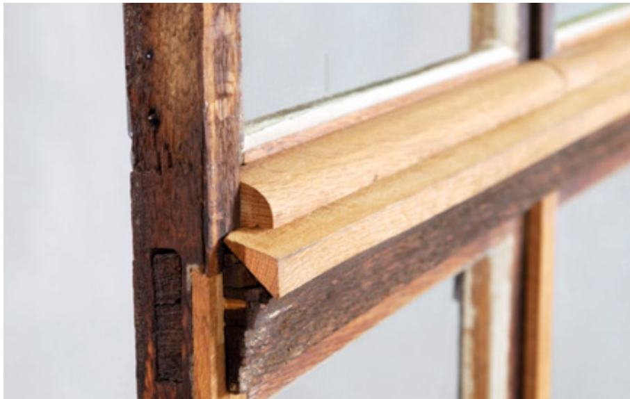
Figure 1: Repair of a window frame, where damaged parts are replaced with the same type of wood, still visibly distinguished by color. Image: Johannes Mosler
