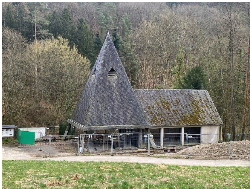
Figure 45: The cemetery chapel in Rhöndorf following initial measures to preserve the structure.
