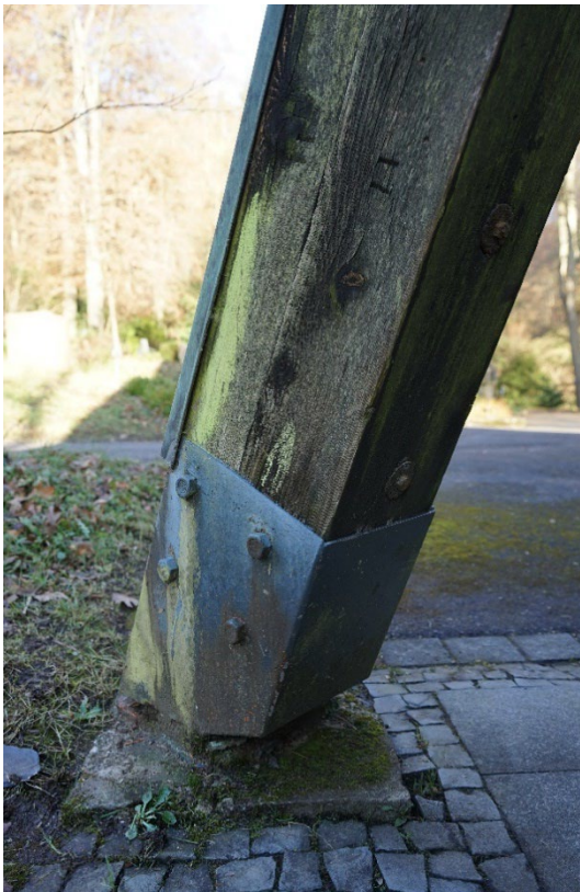
Figure 51: Extensive rot on all four main columns was documented.
