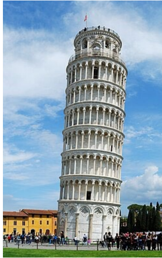
Figure 27: A notable example of a structural flaw that has been kept by intention. Image: Saffron Blaze.
